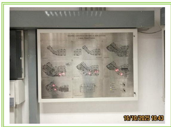
Graphic Annunciator Fire Protection System
